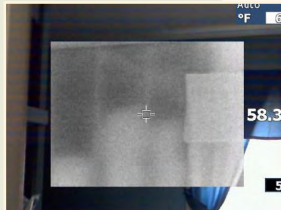
Infrared technology allows weatherization professionals to examine insulation in exterior walls.
