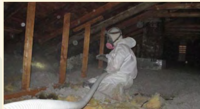
ADVOCAP staff member insulating the attic of a home.
