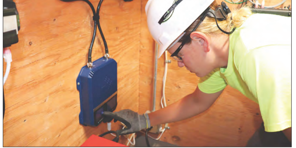
Shea Electric & Communications photo
